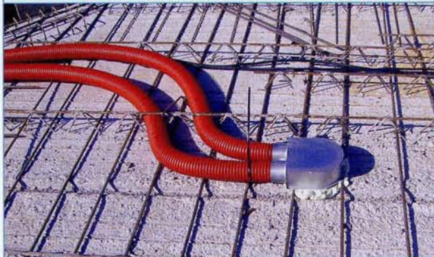
In the concrete ceiling screed
