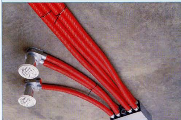
From a suspended ceiling
